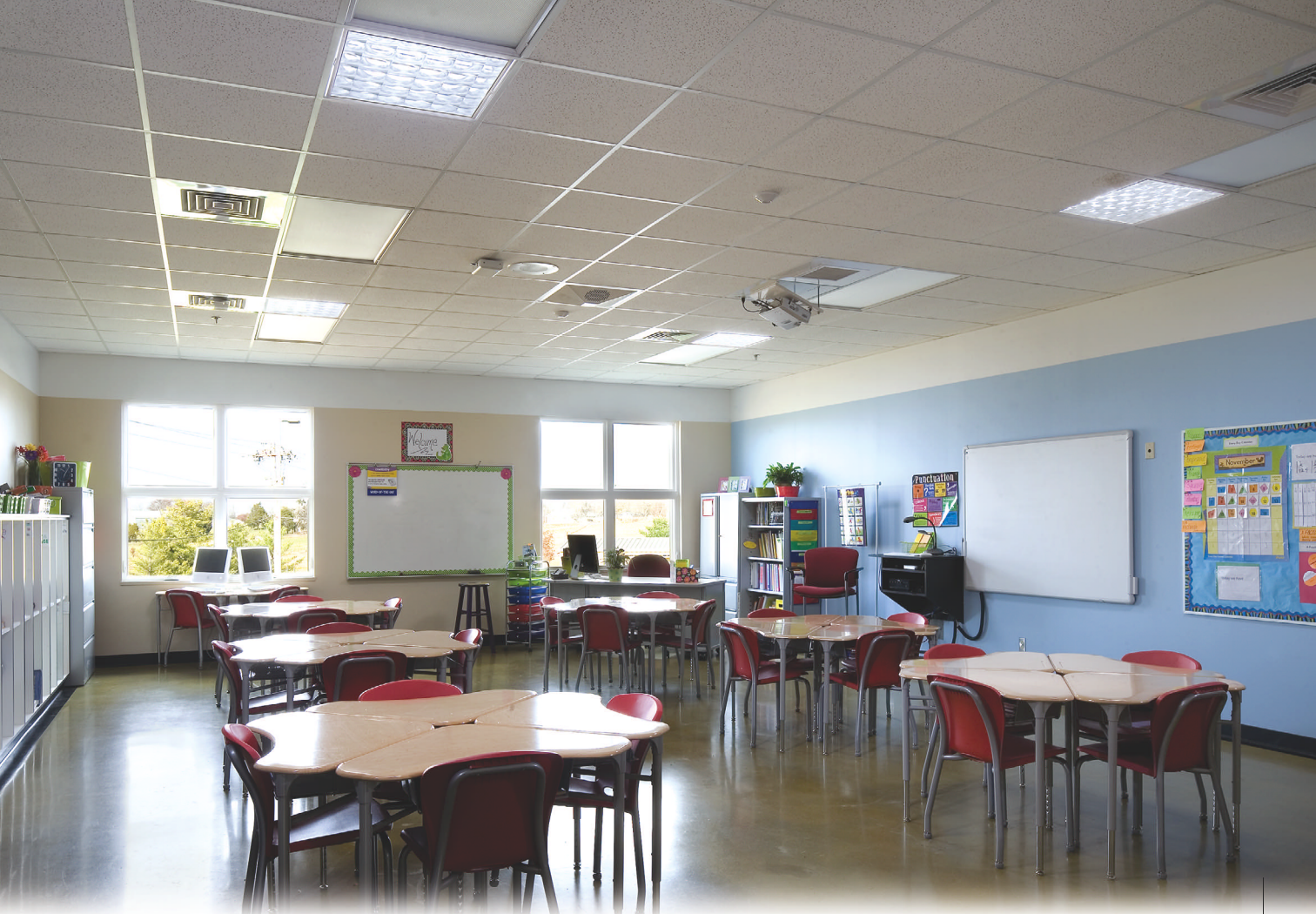
Classrooms on the north-facing side of Richardsville Elementary School have four tubular daylighting devices that provide top-lighting. Courtesy: CMTA, used with permission from Rachel Paul Photography
