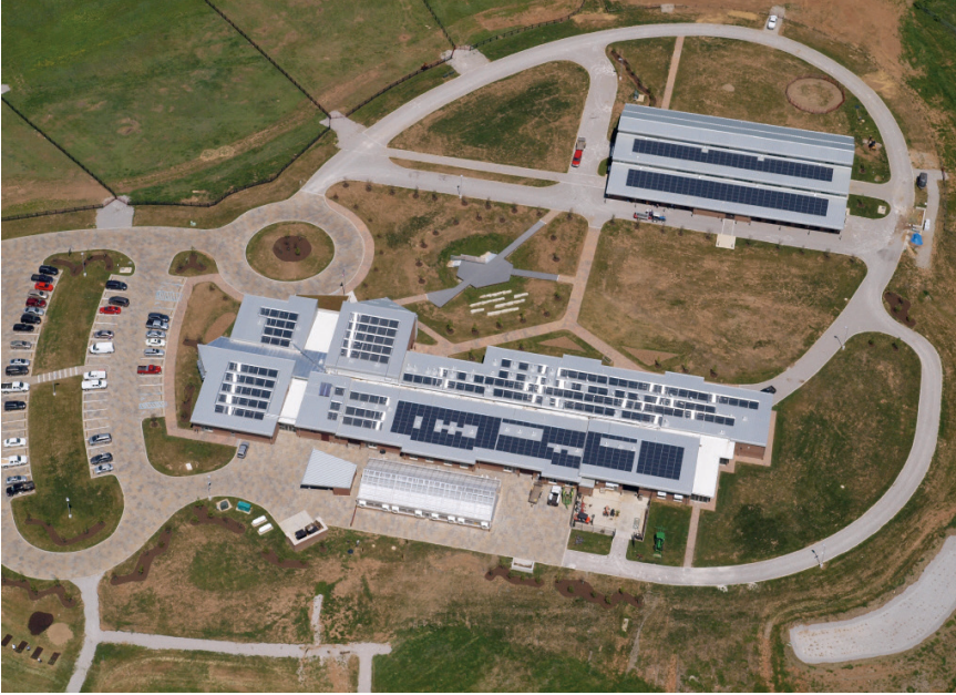
Above An aerial view of Locust Trace AgriScience Center shows (from bottom) the greenhouse, academic building, outdoor teaching space and arena. The building orientations allows for maximum solar exposure for the solar photovoltaic and solar thermal arrays.
