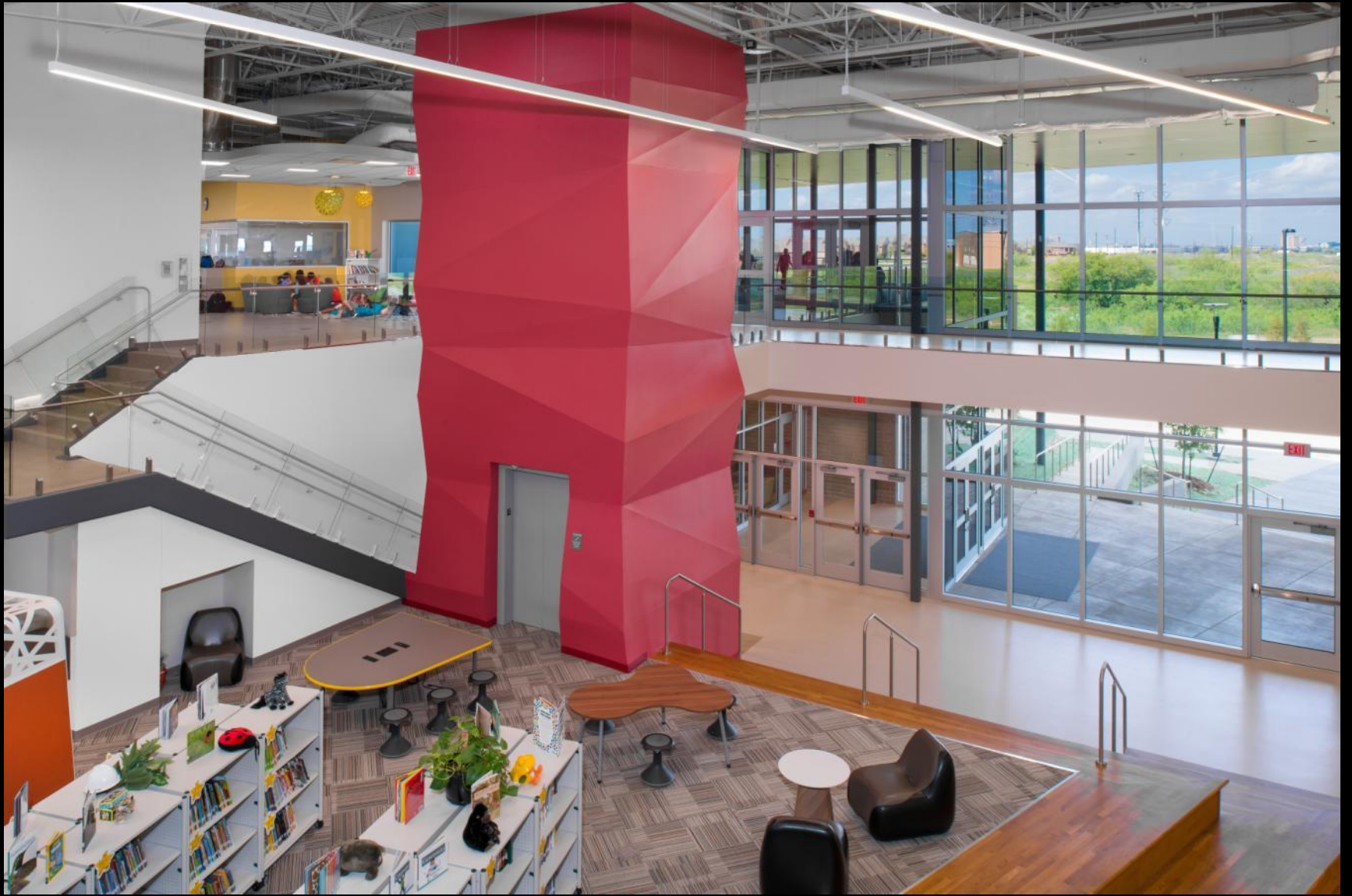
Richard Lee Elementary School, LEED Target - Gold
