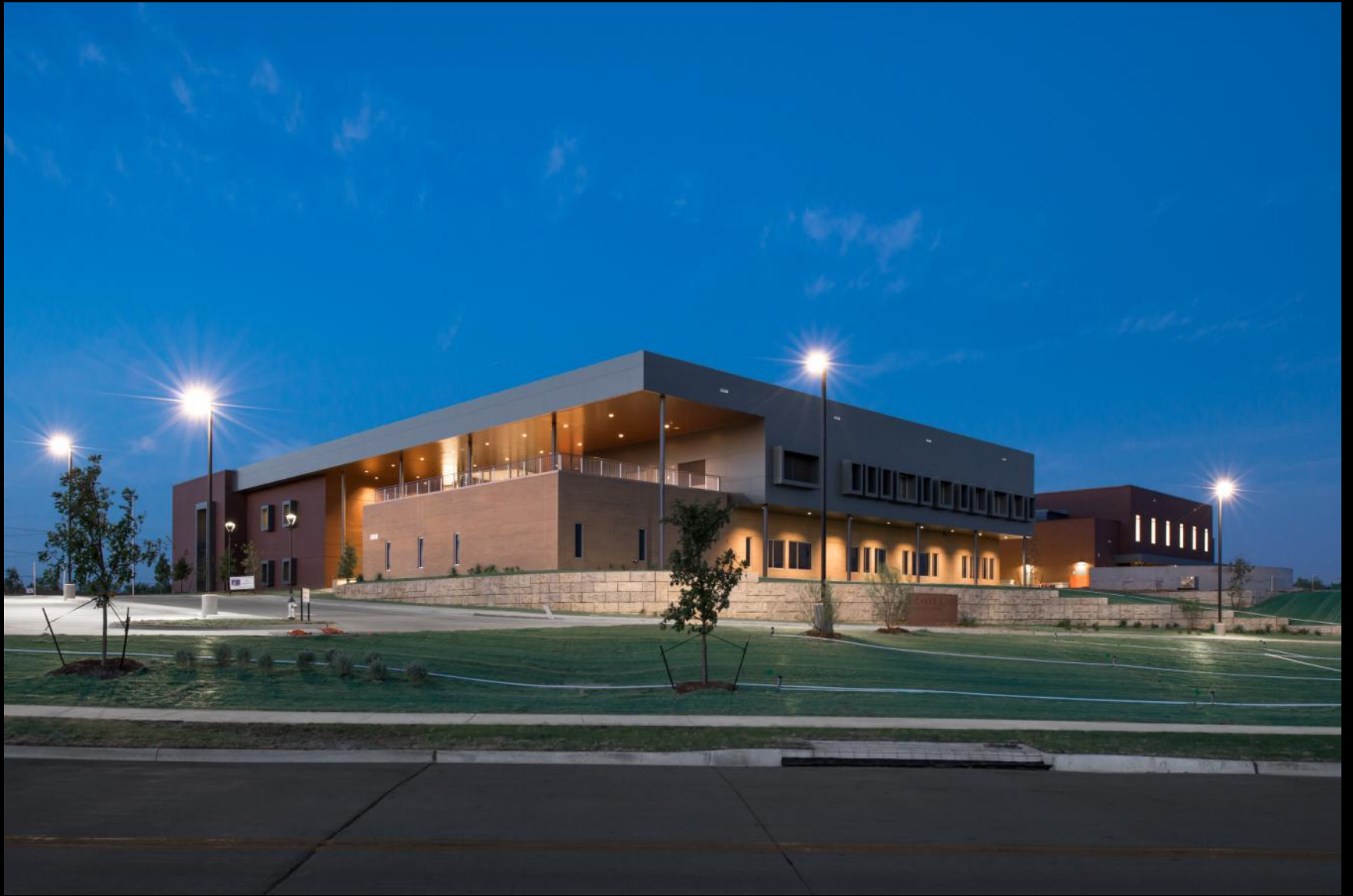
Richard Lee Elementary School, LEED Target - Gold
