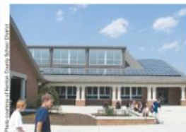
The 22 kW solar photovoltaic array, seen from the front entrance of the school, consists of 26 crystalline silicon PV panels, each rated for 110 watts and configured in four strings that are
