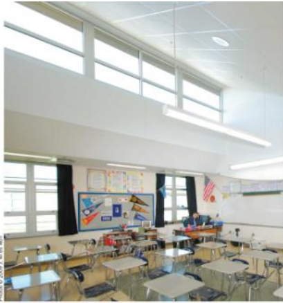
Roof dormer windows provide daylighting in Twenhohel Middle School classrooms. This design provides natural light deeper into the classrooms than some other configurations. Fluorescent lighting systems automatically dim as daylight increases.
