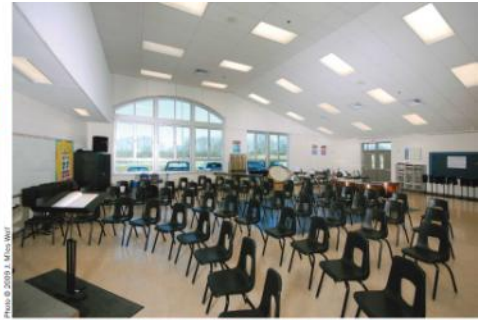
A geothermal heat pump system serves the music room and the rest of Twenhofel Middle School.
