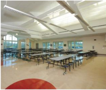
Ceiling baffles (top right) restrict the sunlight in the cafeteria and other south-facing rooms.
