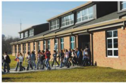
The roof dormer glazing provides natural light to classrooms. After daylighting was successfully implemented at Twenhofel, the Kentucky Department of Education reduced the artificial lighting requirements for daylight classrooms to 40 footcandles.
