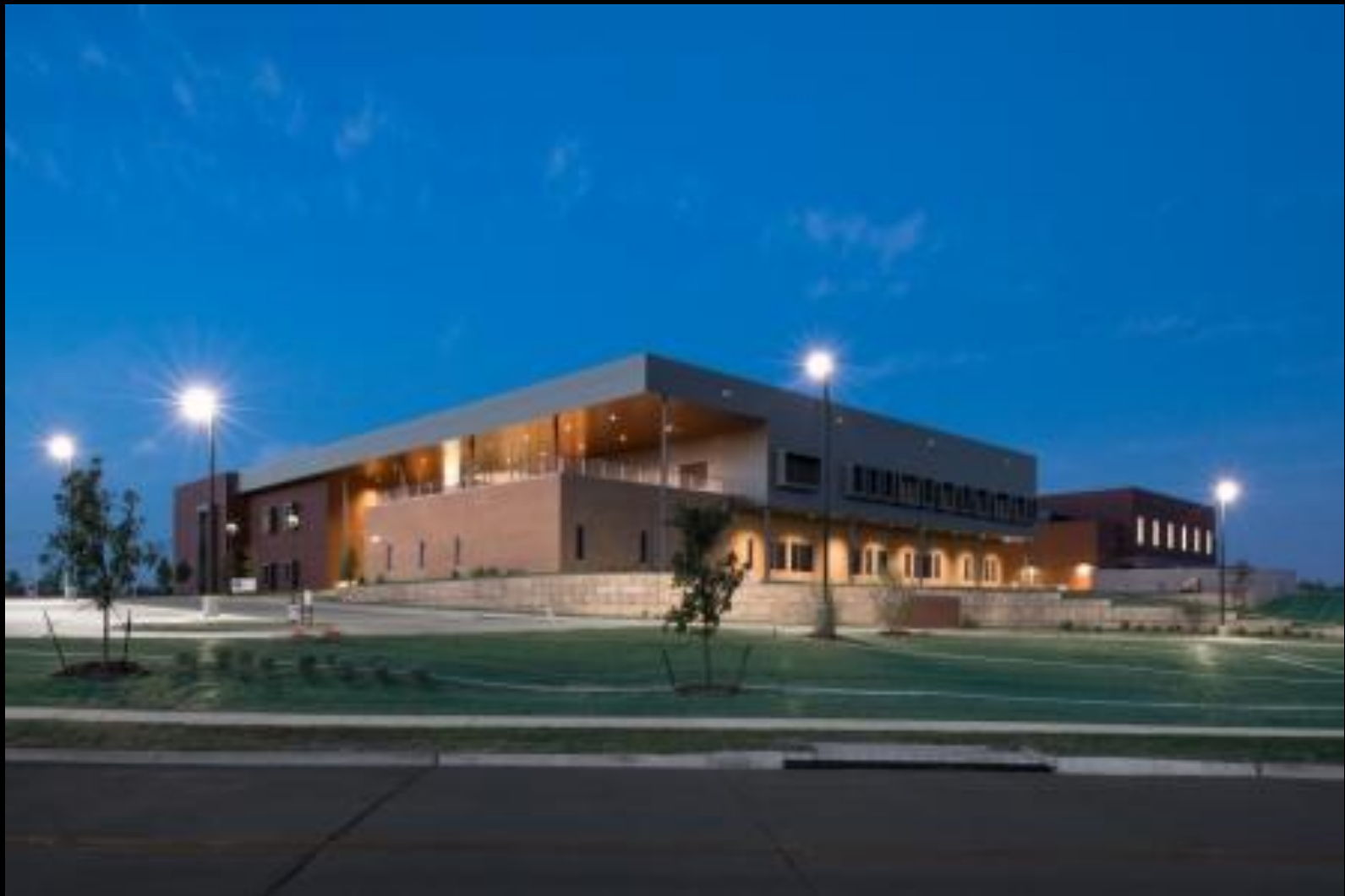
Lee Elementary School – Net Zero Energy School, Dallas, Texas Stantec/CMTA
